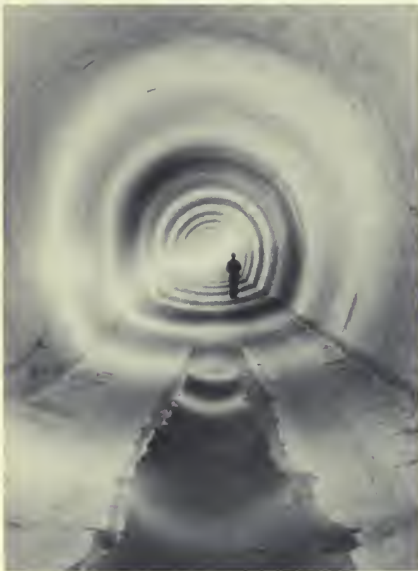
MAN-MADE CAVERN is the Frenchman Hills tunnel, 16 feet in diameter, shown above. Puddle of water inside tunnel, at left, is hardly a forerunner of things to come, when enough water to irrigate 50,000 acres will pour through the structure. All photos by Harold E. Foss, Region 1.
